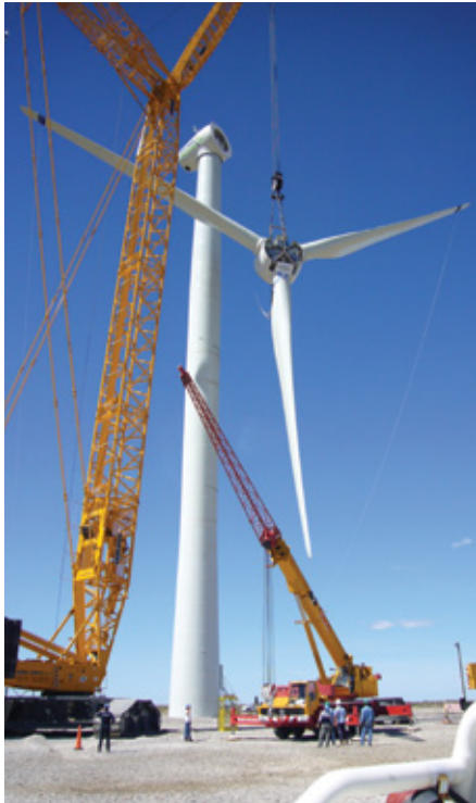
Construction at the El Torcillo Wind Farm in Chubut Province, Argentina
